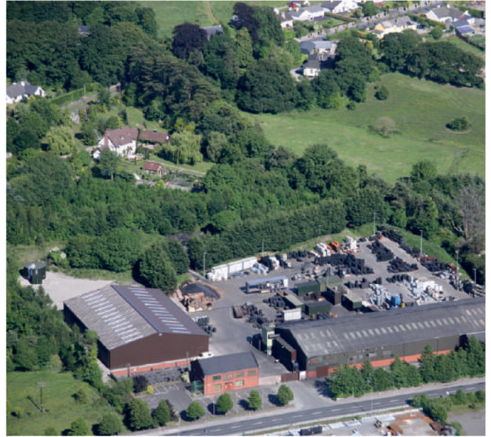
Birr -Ireland , with both a composite production site and a fabricated steel facility. Management system certification includes ISO 9001, ISO 14001 and ISO 45001 for quality management, environment, health and safety.
