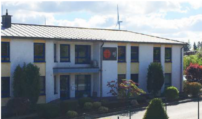
Boppard - Germany - Our production on the Rhine, Germany: a total of 70 employees - development and production of steel and stainless steel solutions. Management system certified according to ISO 9001 for quality management.
