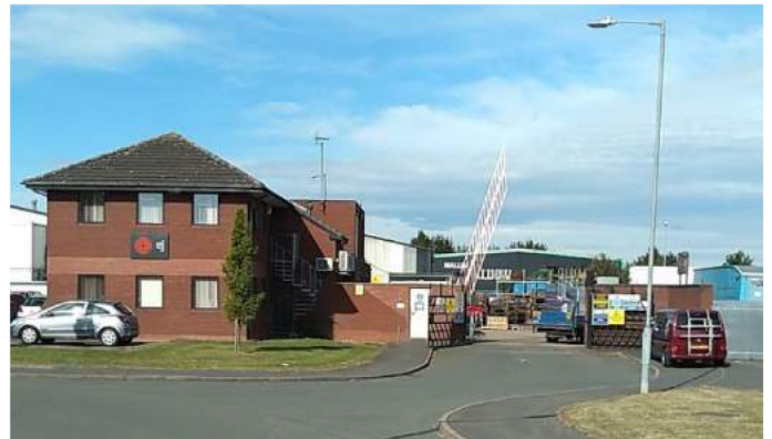
Nuneaton - UK - This is our UK distribution & manufacturing facility for galvanized and stainless steel products. Our UK facility is certified to ISO 9001 for quality management and ISO 14001 for environmental management.
